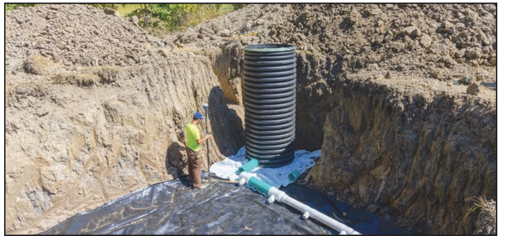
Filters like this one in Defiance County remove phosphorus from farm runoff. They're part of a broader effort to reduce harmful algal blooms in Lake Erie
