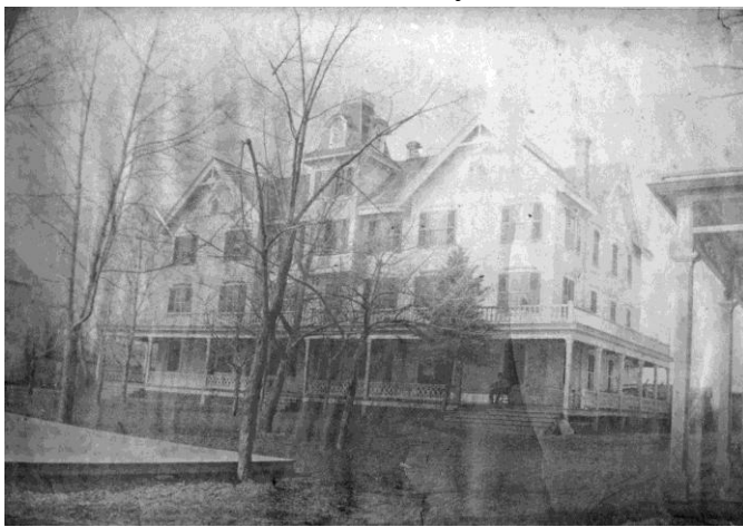
The Himmelein House
