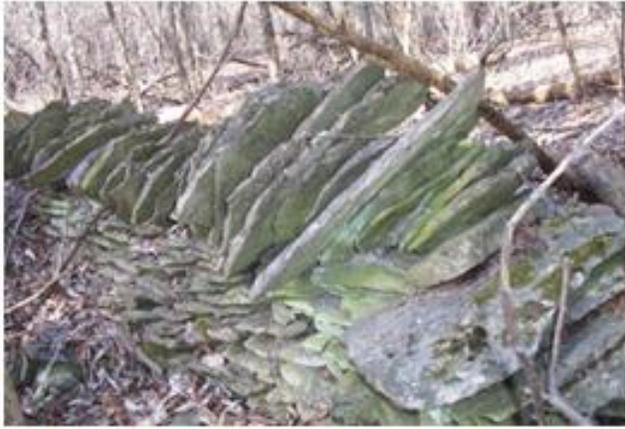
There was a lot of variety in the construction of stone fences, with changes in the top stones marking a boundary change. Sometimes, as with the Long Point fence, large round stones, probably driven onto the land by wave action were incorporated into the design, while inland fences tended to have just flat stones.
