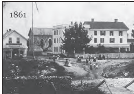
The telegraph would be located in Huntington's Store (The Store on the Corner or more commonly known as The Lodge), which was also the Post Office (the small building on the left).
